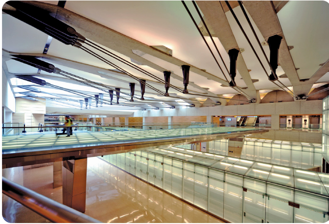
Dulles International Airport Automated People Mover
