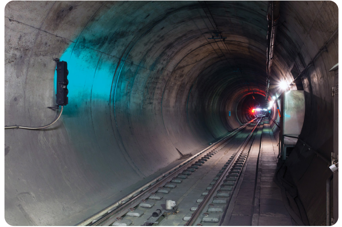
Dallas Area Rapid Transit Tunnels and Station
