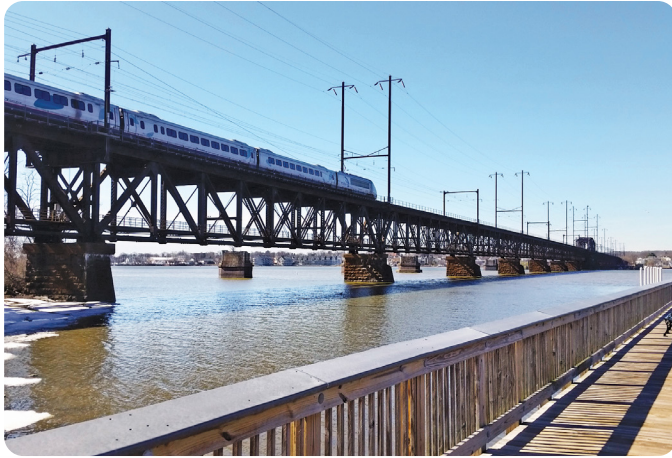
Amtrak Susquehanna River Rail Bridge
