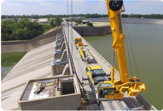
Canton Dam Gate Replacement
