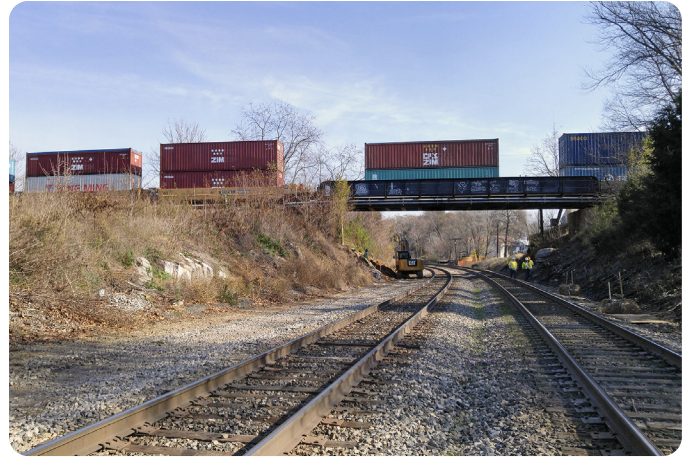
CSX National Gateway Phase 2
