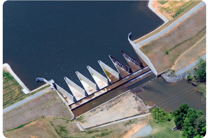
Lake Townsend Dam
