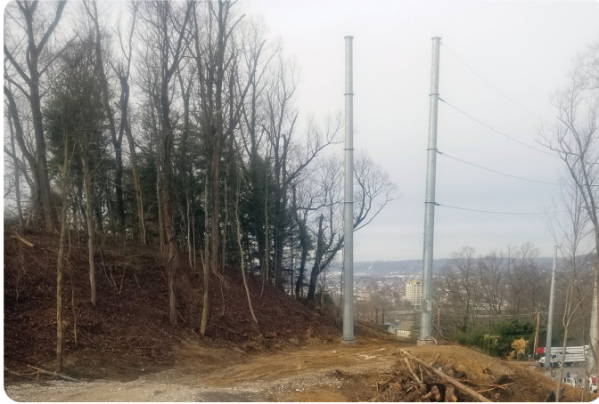
AEP Bullitt Street Chesterfield Avenue 138 kV Line Replacement
