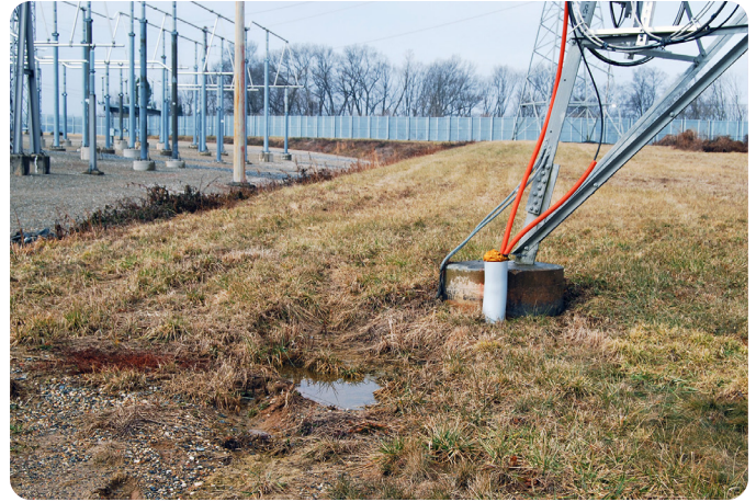
Baltimore Gas & Electric 230 kV Conastone to Northeast Rebuild
