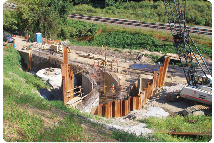
Battery Park Trunk Sewer Emergency Tunnel
