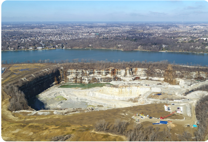
Quarry Conversion to Citizens Reservoir
