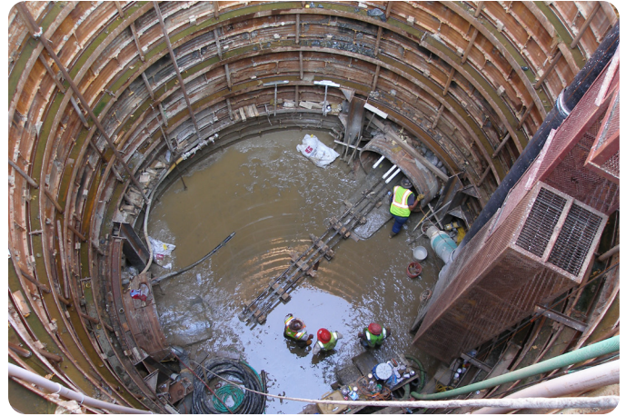
Greensferry Sewer Tunnel
