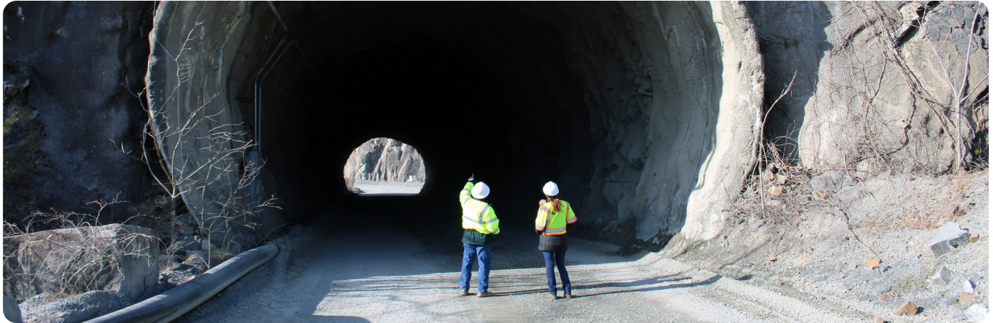
Quarry A Pumped Water Storage Reservoir
