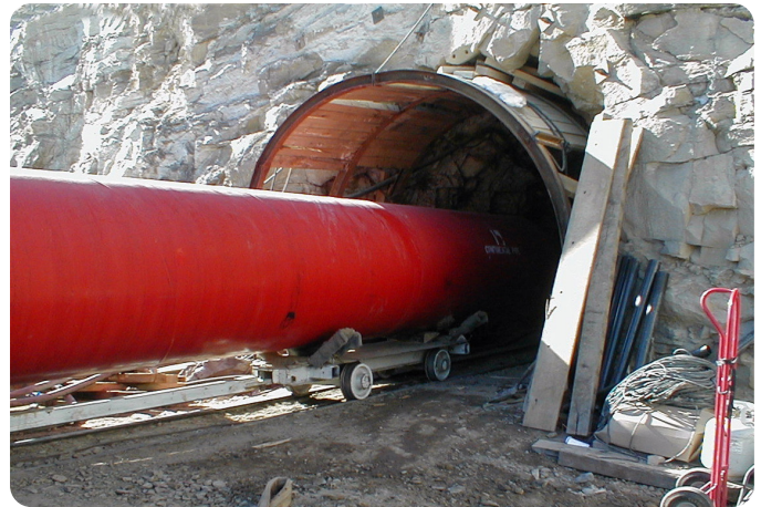
Plateau Creek Pipeline Tunnels
