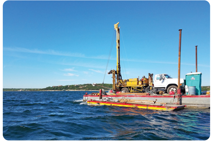
BCRUA Deep Water Intake Project, Phase 2
