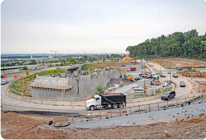
DDOT I-295 / Malcolm X Avenue Interchange
