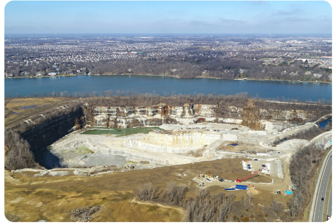
Quarry Conversion to Citizens Reservoir
