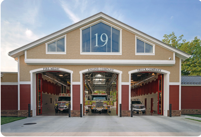
Henrico County Fire Station No. 19
