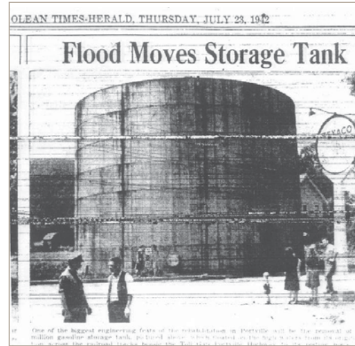
In 1942, rainfall in Smethport, Pennsylvania was estimated to be nearly 31 inches in less than 5 hours. This estimate exceeds the hypothetical PMP. The flood waters picked up and moved this water tank well downstream.
