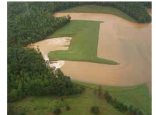
Rainfall from storms in Georgia in September 2009 was estimated to exceed 50 percent of the PMP, causing activation of auxiliary spillways like these at Snake Creek Dam.
