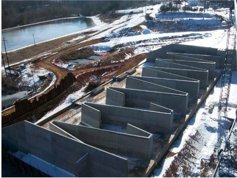
Fig. 1 – Photograph of the construction of the 7-cycle labyrinth spillway at Lake Townsend (North Carolina, USA)
