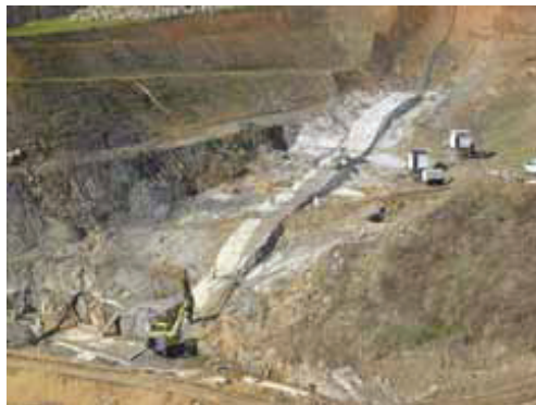
Rocky Pen Run Foundation Grout Curtain Stafford County, Virginia
