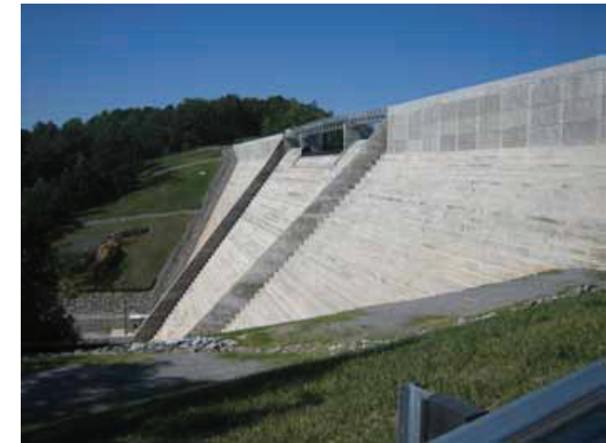
Hickory Log Dam, Canton, Georgia
