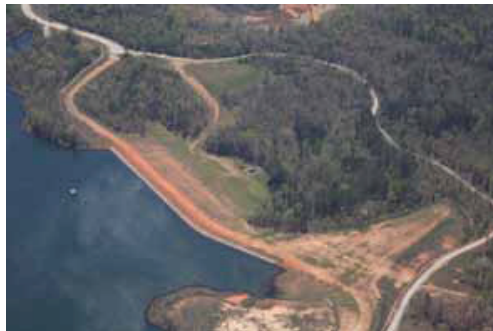
Cedar Creek Dam, Hall County, Georgia
