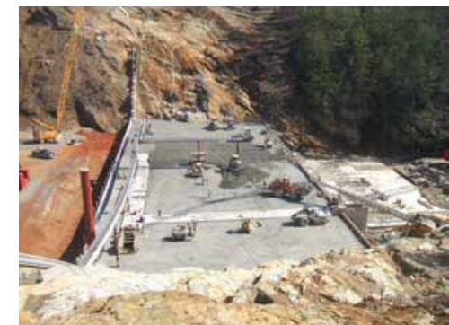
Early Construction, Hickory Log Dam Canton, Georgia
